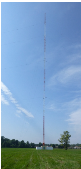
Here's a picture of a Michigan AM tower. Photo Credit: http://www.michiganbroadcasttowers.com/towers/sea03.html
